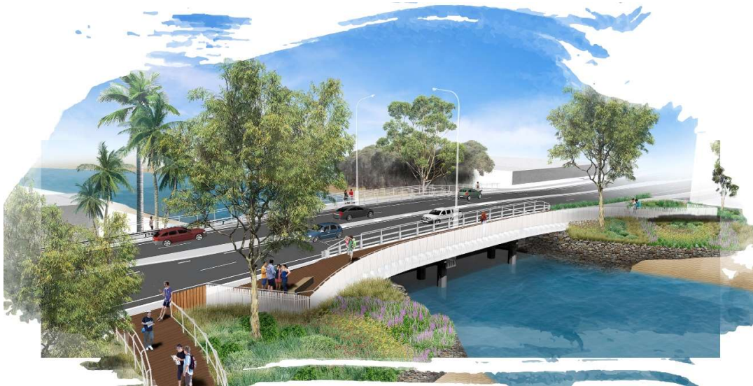
Figure 2. Artist impression of new, four lane Mayes Canal Bridge featuring timber decking and a shared pedestrian and cycle path on both sides of the bridge.
