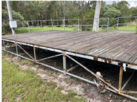
Stage & Retaining Wall
