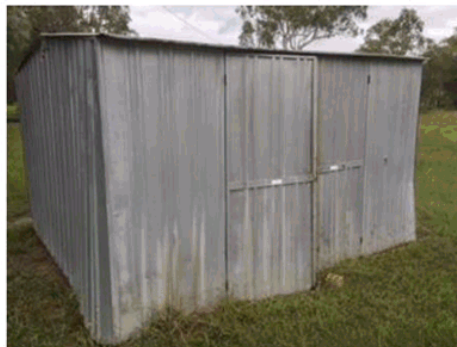
Bore & Pump Shed
