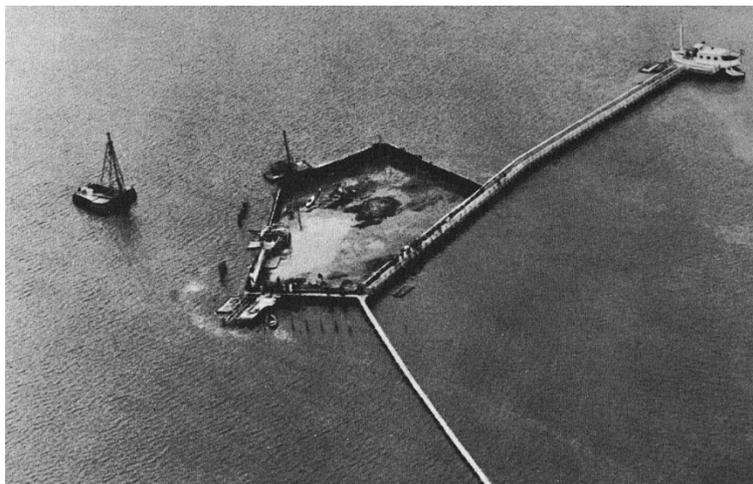
**Figure 50. Cofferdam in Roskilde Fjord constructed during 1962 for excavation and recovery of five Viking ships.<sup>134</sup>**
