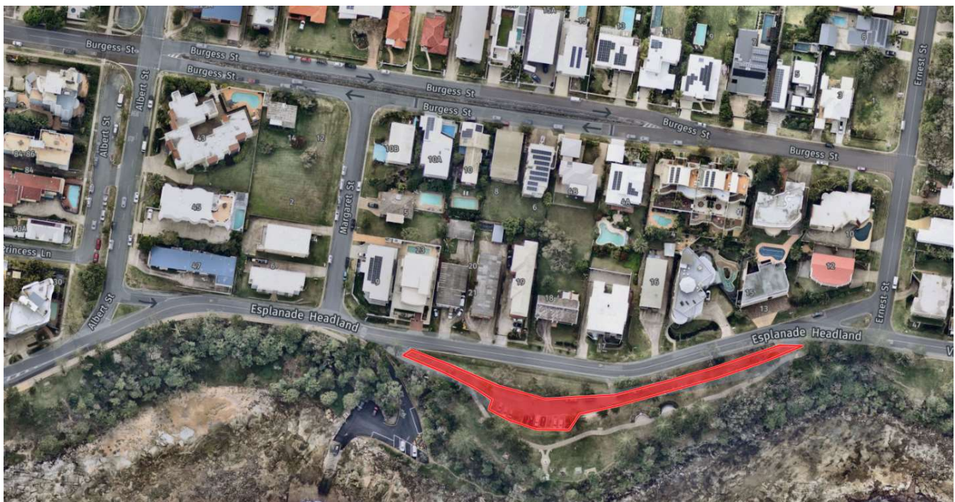
Figure 2. Centaur Park access road and car park temporary closure – estimated to remain in place until 30 June 2024 (during construction)
