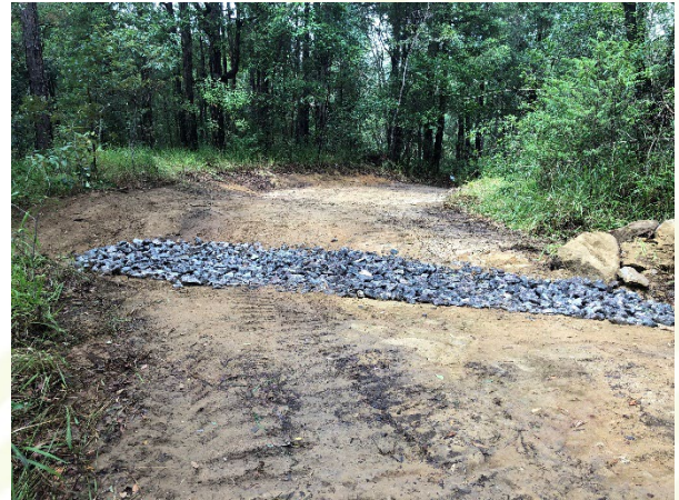
A rock swale drain in an erosion-prone area.
