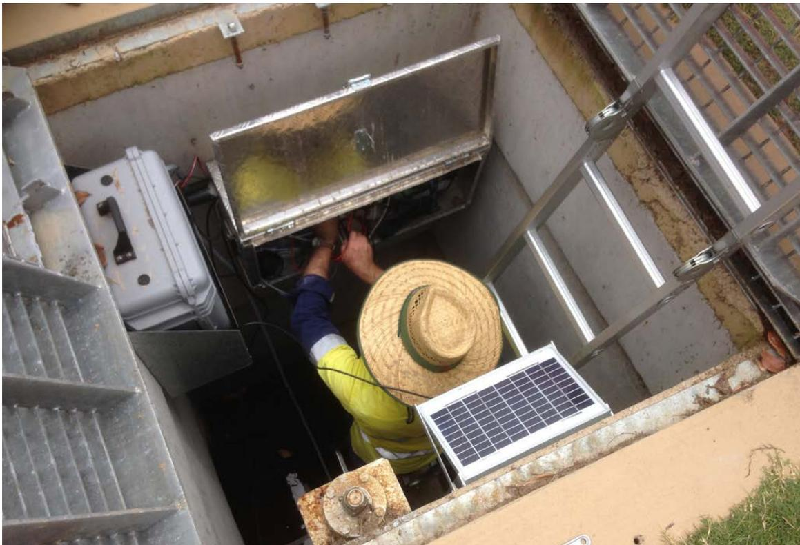
*Figure 3 – Installation of Automated Water Sampling Equipment in Diversion Pit*
