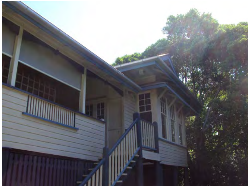
Photo: Wallace House, front stairs and verandah, 2012
