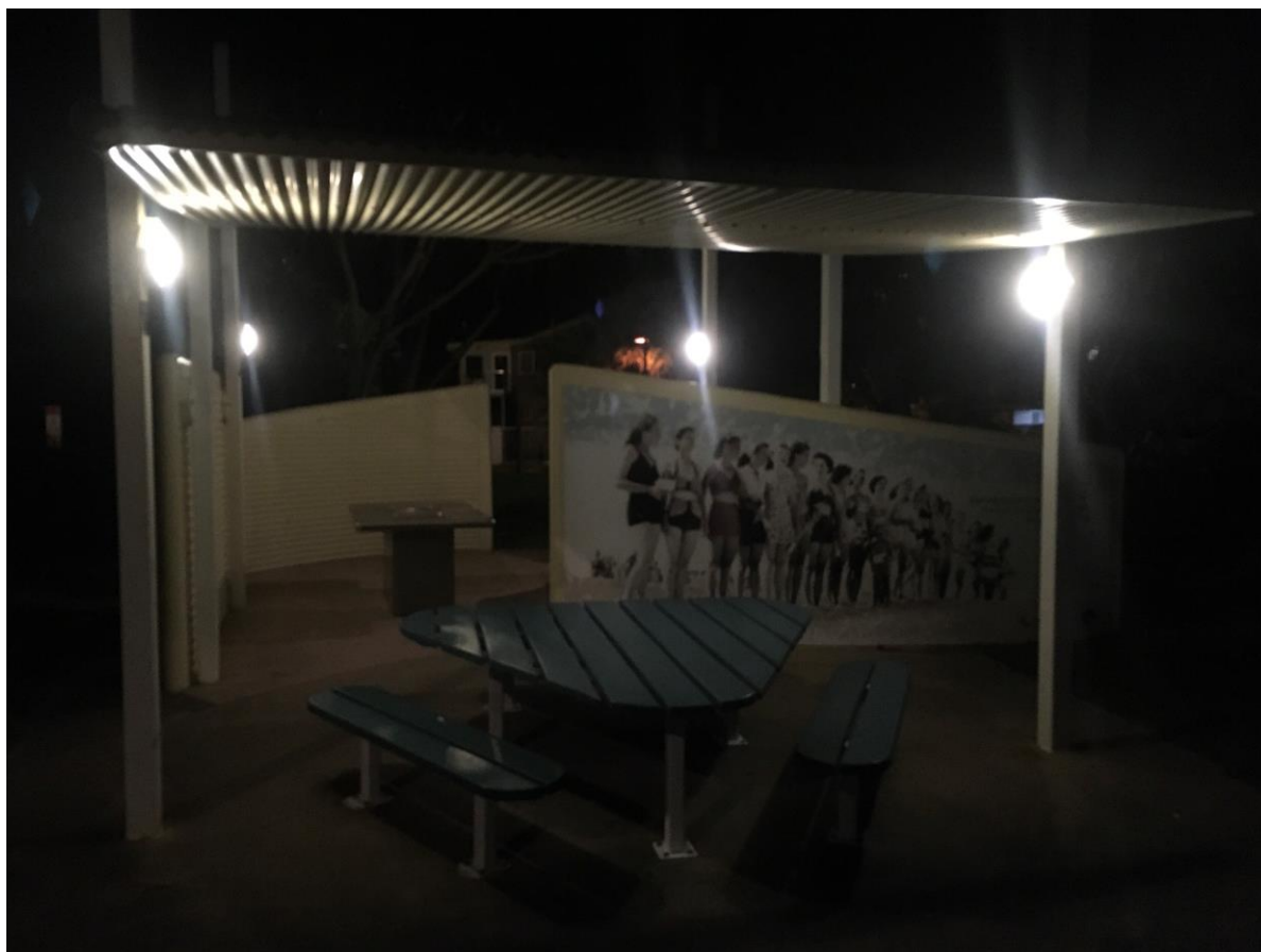
Image 26: Light sources mounted on poles of picnic shelters produce significant spill light and only a small portion of the light output is used for the intended purpose. Recessed light fittings, or light fittings with cut-off reflectors or sides, are useful to reduce spill light and its contribution to sky glow.
