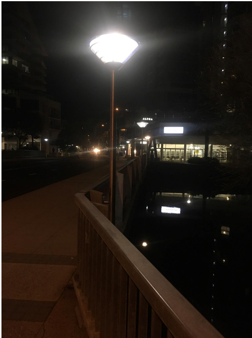
Image 37: Bridge lighting uses diffuse sources which spread the light beyond the intended area and into the waters below.
