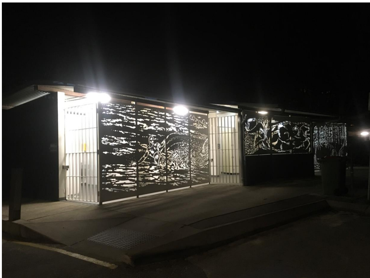
Image 28: Amenity blocks produce significant spill light, including at times when they are locked and not in use. Amenity blocks often utilise surface mounted, diffuse, linear battens which produce light beyond the intended area. Dimmers, motion sensors, and timers are useful for only illuminating the area when required and to the level required.
