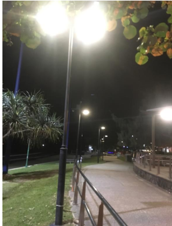
Image 36: Footpath lighting in Mooloolaba Foreshore Park illuminates larger areas than required and spills light onto the beach.
