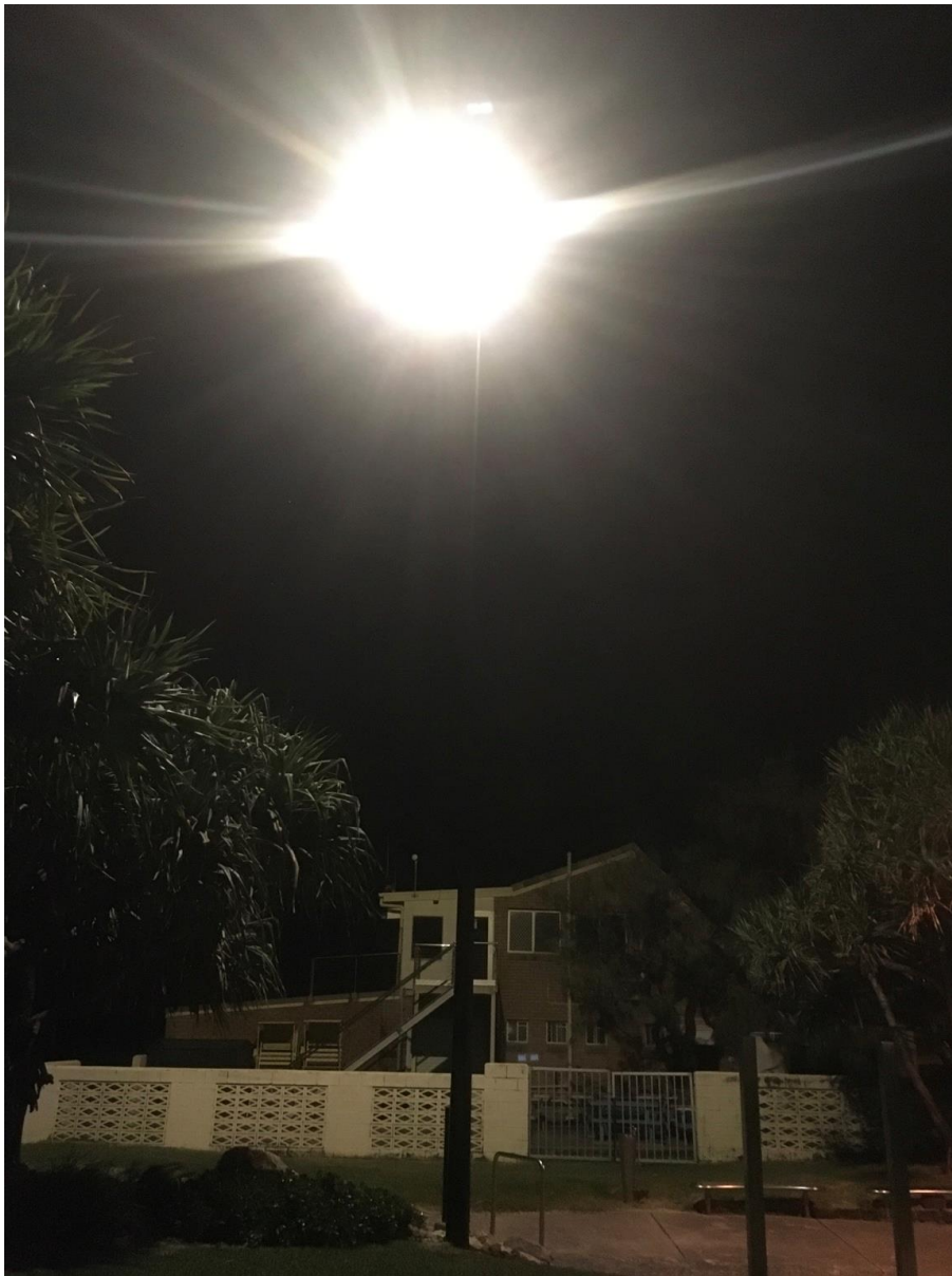
Image 31: High mounted park lighting illuminate properties beyond the intended area, and are visible from the beach.
