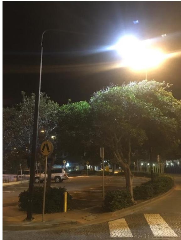
Image 23: Multiple light sources illuminating vegetation and casting shadows on a pedestrian crossing, road and carpark – the areas intended for illumination. Light sources mounted below the tree line that illuminate only the intended area would reduce energy consumption and sky glow.
