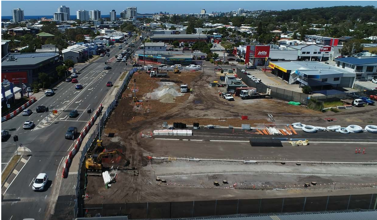
Figure 6. Aerodrome Road Intersection Works
