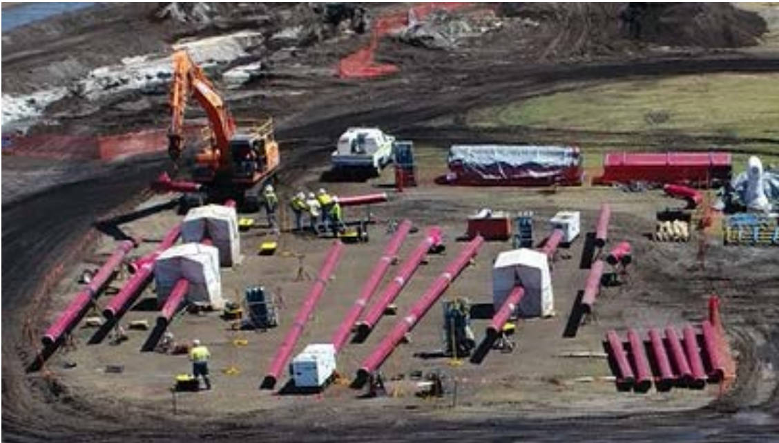
Figure 4. Stage 1A – AWCS Pipe Preparations
