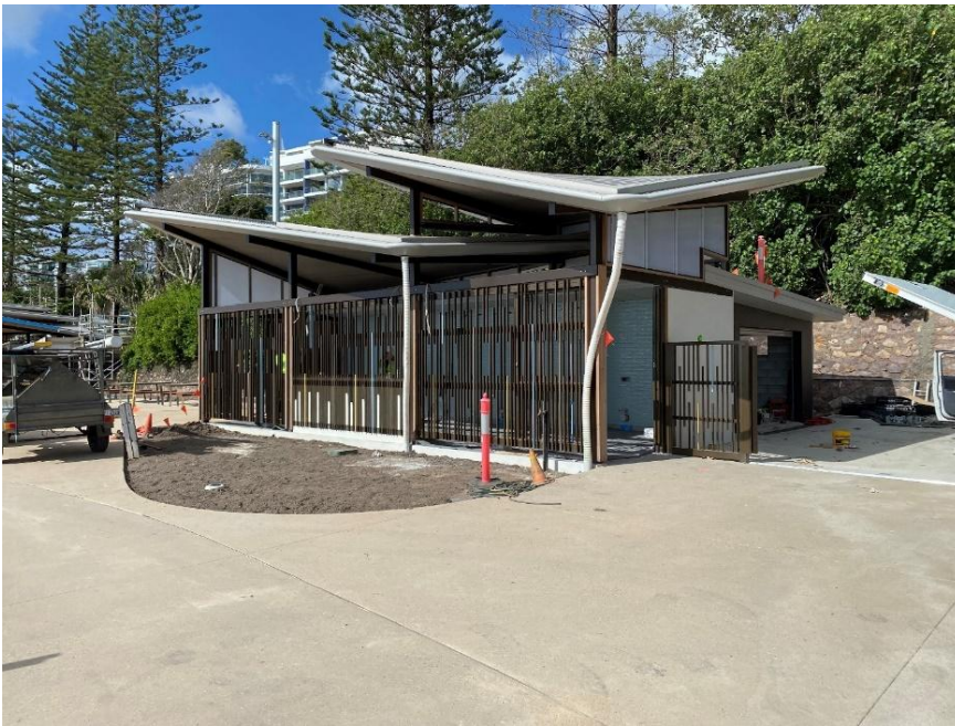
Figure 2 New public amenities building in the Northern Parkland - landscaping to come
