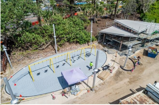
Figure 1 New swing set being installed prior to shade sail installation
