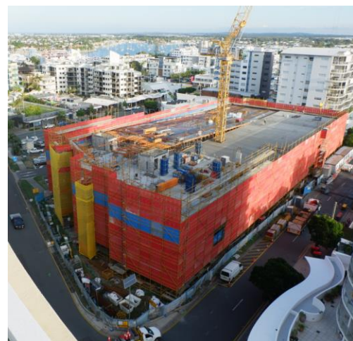
Multi-deck car park, June 15 2020
