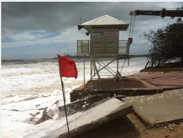
Figure 1 Mooloolaba Surf Life Saving tower damage from Ex-Tropical Cycle Oswald in January 2013.
