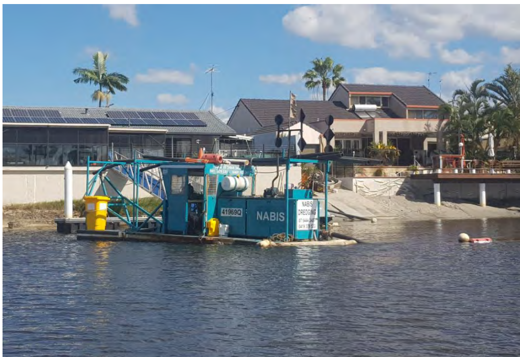
Figure 3-3 Dredging in progress to raise canal beach levels
