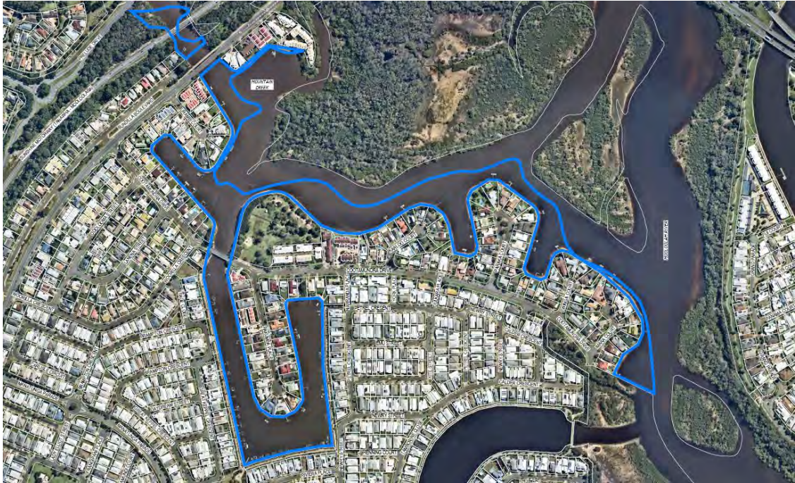
Figure 2-4 Hideaway Waters Canal System
