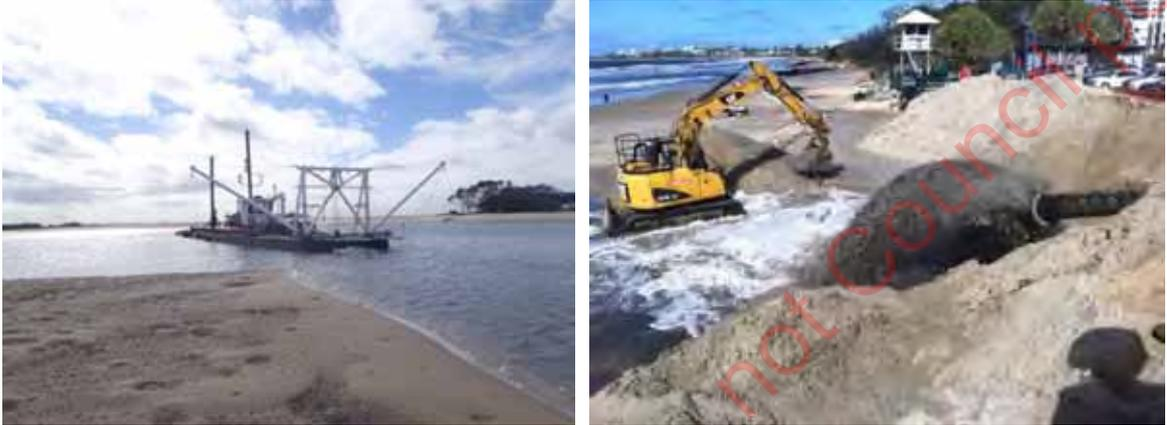
**Figure 2-20 Cutter Suction Dredge and Pipeline Sand Delivery to Maroochy Beach**
