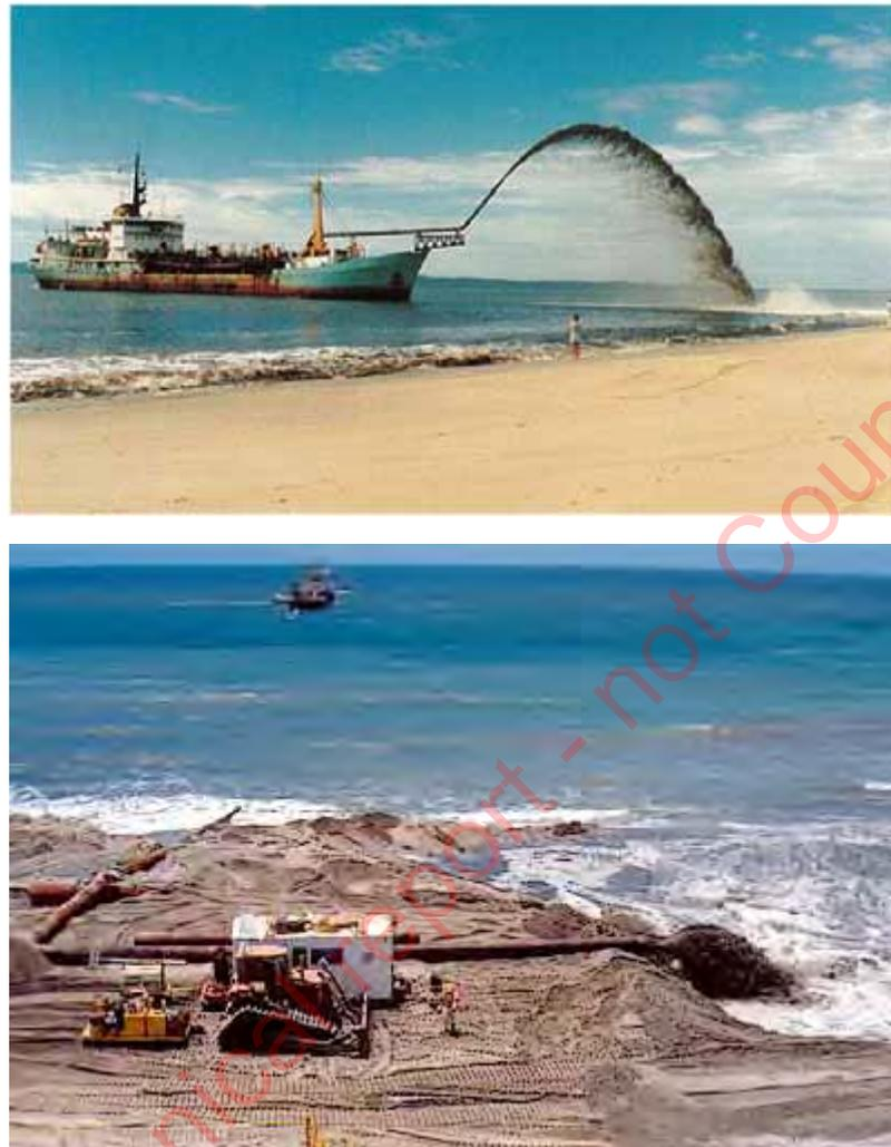
Figure 2-7 Rainbowing at Woorim Beach (top panel, BMT WBM, 2014) and Pumping Sand Onshore (bottom panel, SANDAG, 2015)
