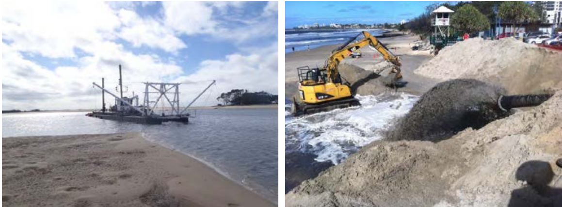
Figure 4-3 Cutter Suction Dredge and Pipeline Sand Delivery to Maroochydore Beach
