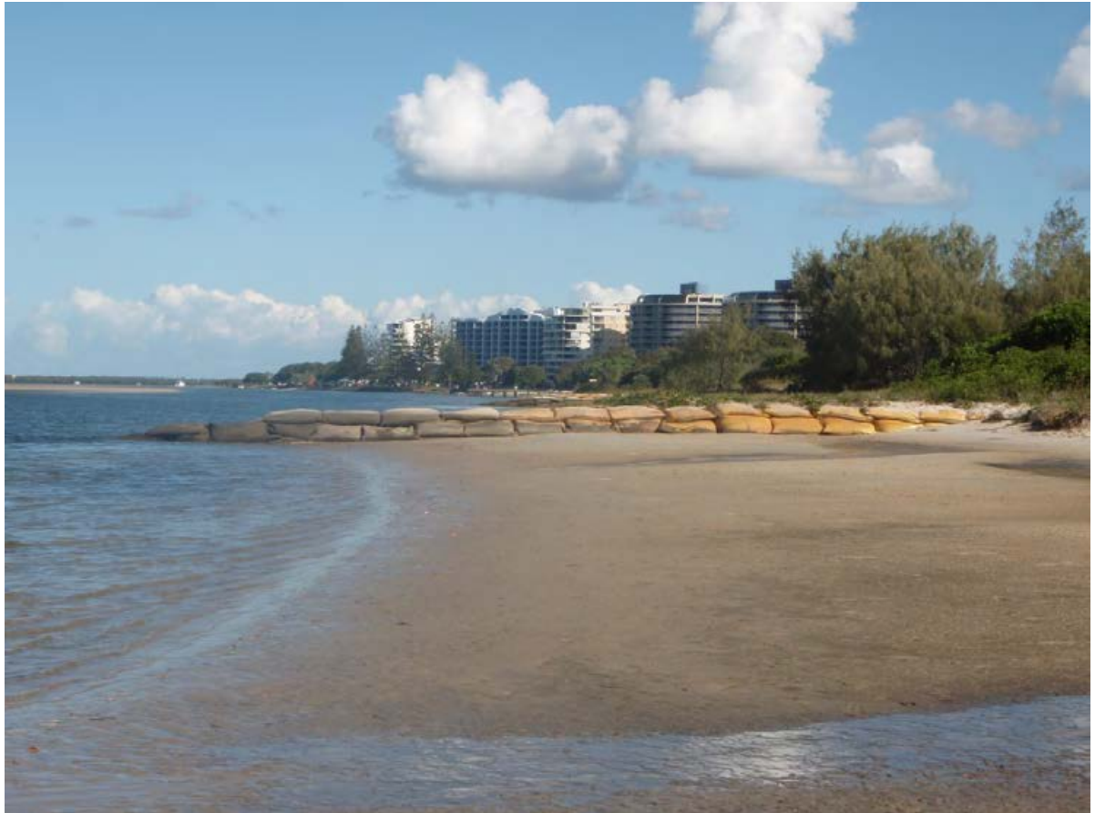
Figure 4-10 Stormwater Outlet Concealed and Protected using Geotextile Sand Containers
