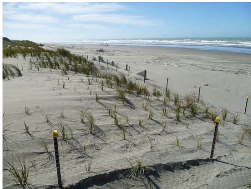
Figure 4-5 Dune Stabilisation using Vegetation and Temporary Access Restriction
