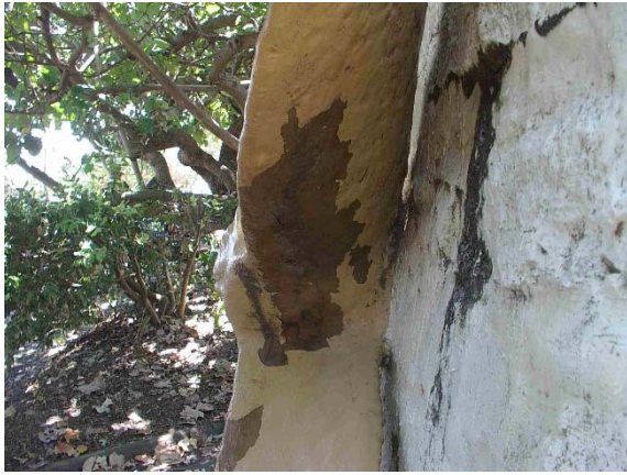
Figure 23. Detail of the layers of fibreglass coating for the propeller at Dicky Beach Carpark. (Cosmos Archaeology, October 2007)
