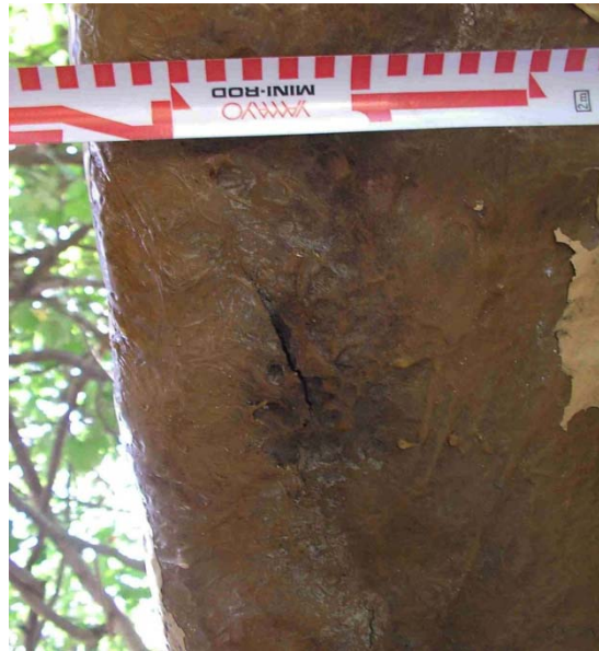
Figure 24. Crack in the fibreglass coating for the propeller at Dicky Beach Carpark. (Cosmos Archaeology, October 2007)
