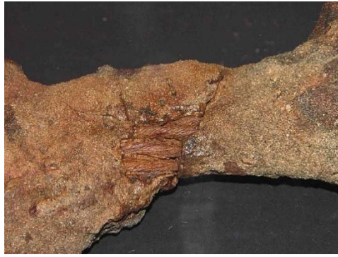
Figure 20. Close up of the steel cable under glass at the Dicky Beach Surf Club (Cosmos Archaeology, October 2007).
