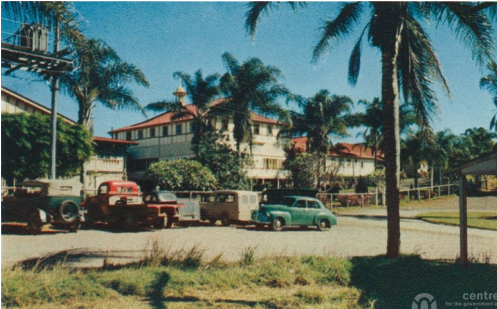
Figure 96: Section of the Nambour Hospital, c1958 (Centre for the Government of Queensland).
