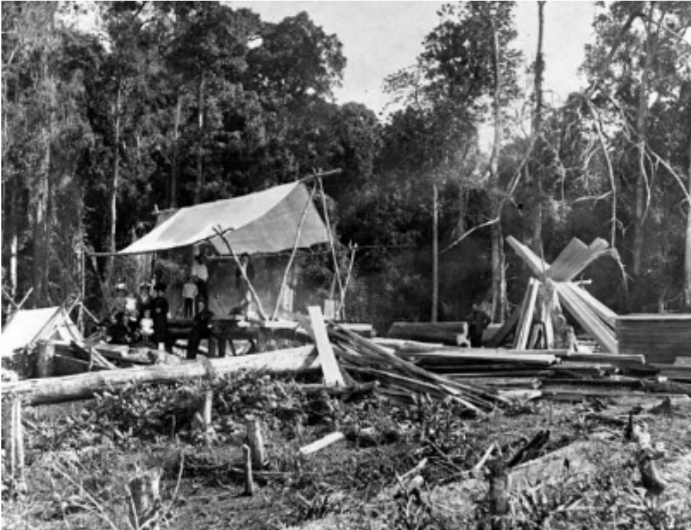
Figure 3: Saw pit in Maleny area c1910 (Sunshine Coast Library).
