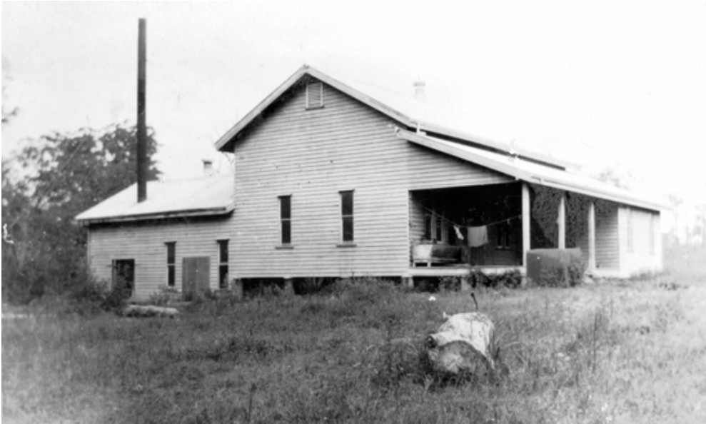
Figure 79: Conondale Butter Factory, 1926 (Sunshine Coast Council Library).
