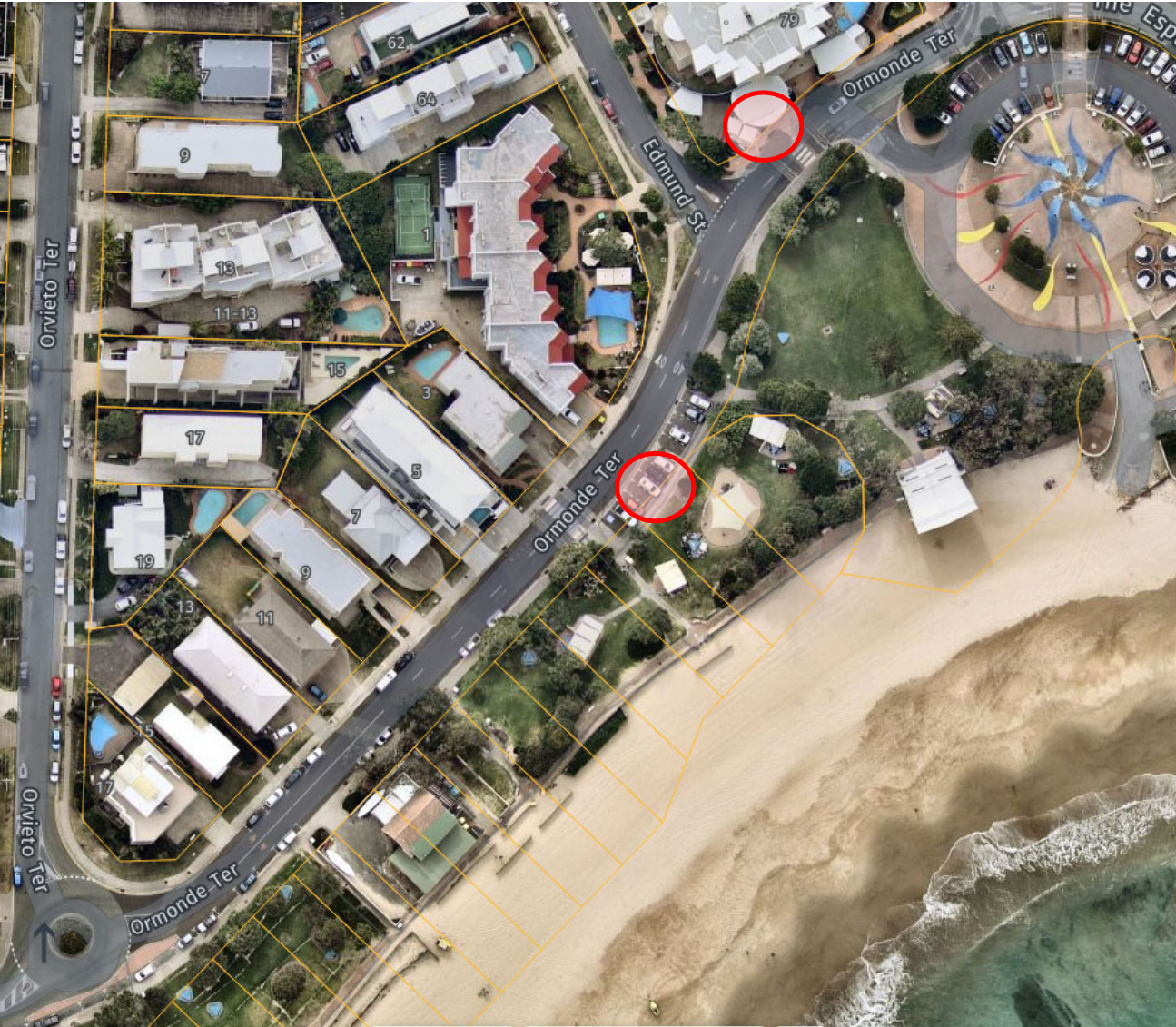
Figure 1: Ormonde Terrace Stormwater Pit Replacement Location
