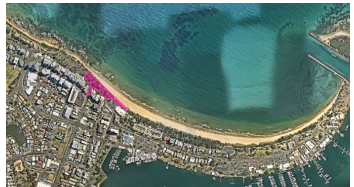
Aerial image of Mooloolaba showing Stage Two works area.
