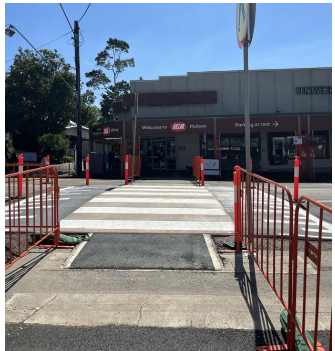
Crossing 4 - now open for pedestrians
