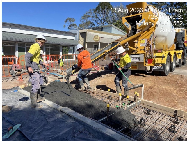
Crossing 1 - under construction
