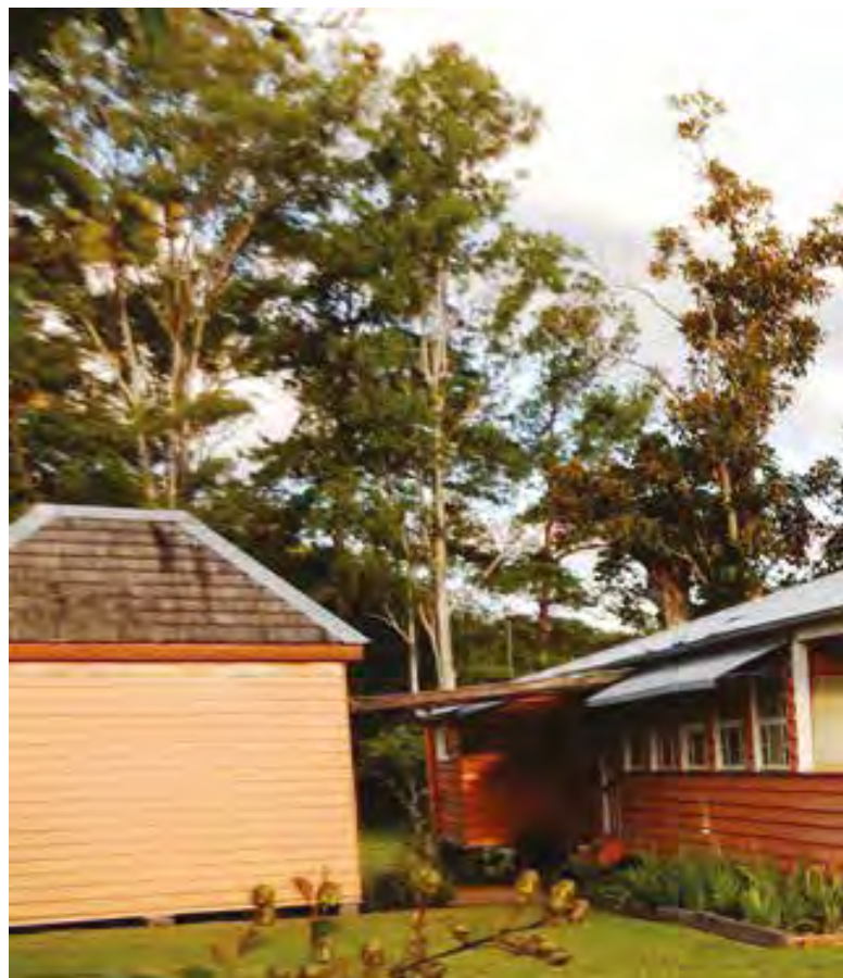
Bankfoot House, Glass House Mountains (current)
